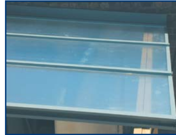
3/ LAY ONTO KERB
