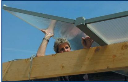
2/ SLOT IN GLAZING PANEL
