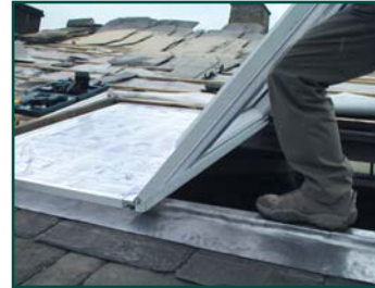
3/ LAY ONTO KERB
